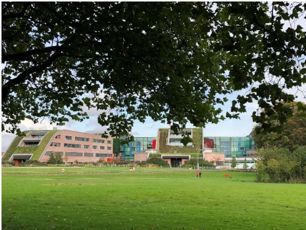
Above: The new hospital buildings have been designed so that children in the wards and their visitors can access garden space. Viewing areas ensure that children who are unable to go outdoors can have sight of green space. Some of the walls of the buildings are also living walls, incorporating plants and greenery.
